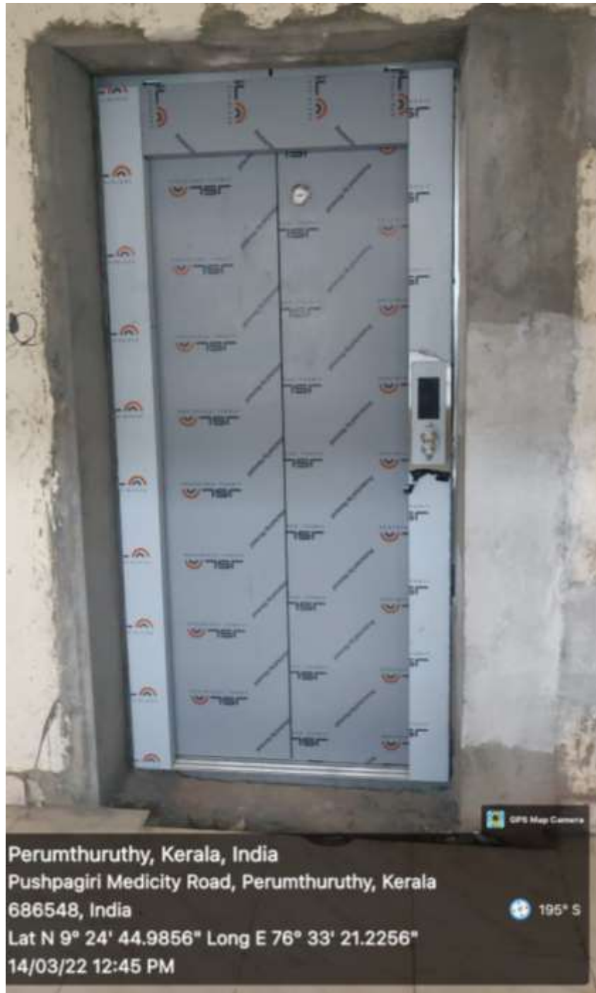
LIFT #2: UNDER CONSTRUCTION
